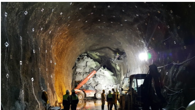
From the Kargi Tunnel repair project in Turkey.
